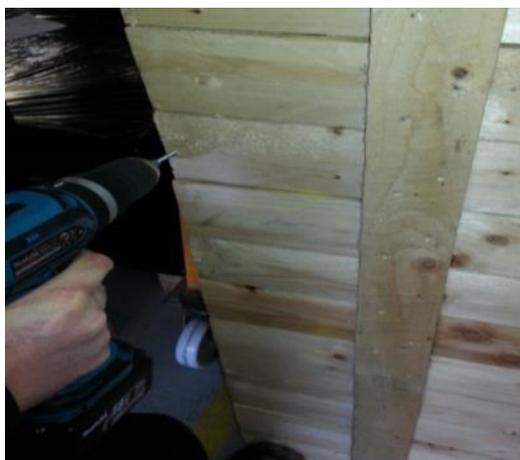
Using a power tool or screw driver remove the screws
