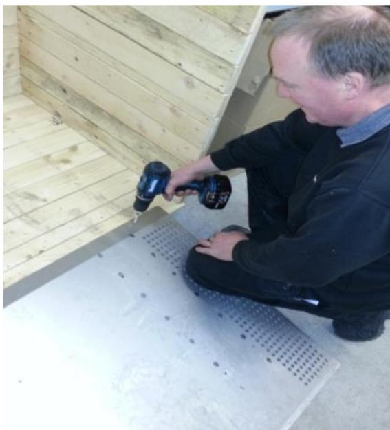
Fix the metal ramp to the wooden container with screws using a power tool or screw driver.
